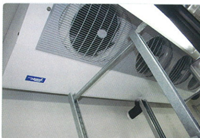
The new LU-VE unit cooler within the freezer case behind the TGD doors is a hitec LU-VE 8 kW SMA 242
