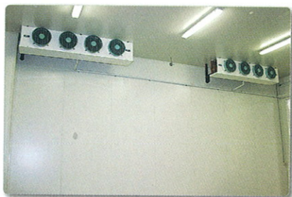
The main produce coolroom with two 16 kW LU-VE S3HC 430 N50 Unit Coolers
