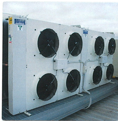
The two 110 kW LU-VE SHVN 110 condensers
