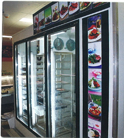
The three TGD doors with top and side mullion illumination
