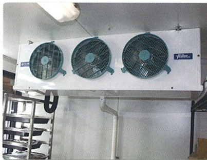
The LU-VE 34 kW S2HC107 N50 Unit cooler in the coolroom behind the TGD doors
