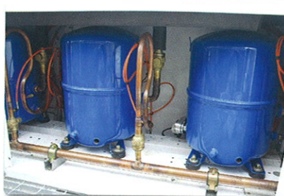
Three 23 kW MTZ 160 Maneurop reciprocation compressors
