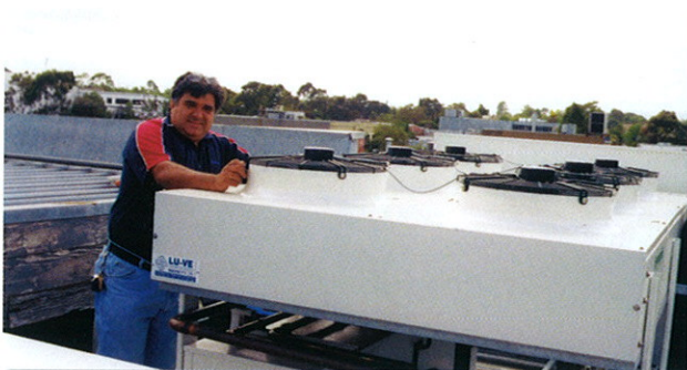
LU-VE's John Mignano with the plug and play refrigeration rack and the SHVN 165 Air Cooled Condenser
